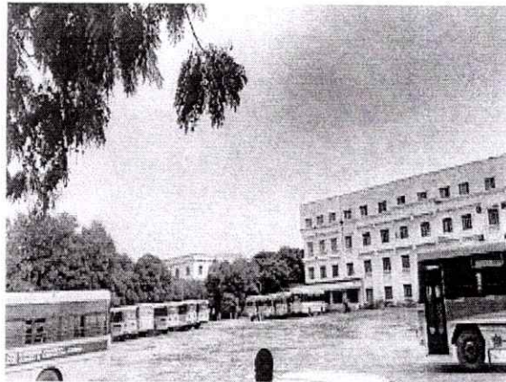
Bus Parking - Near Block-3
