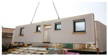
Modular and prefabricated construction are both off-site construction methods that involve building components in a factory or warehouse and then transporting them to the construction site for assembly:
