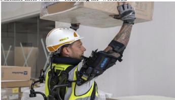
The use of machines such as robots and exoskeletons is another emerging trend in civil engineering. Not only do they resolve mundane tasks with ease, but they also help increase safety and autonomy on-site during construction.
