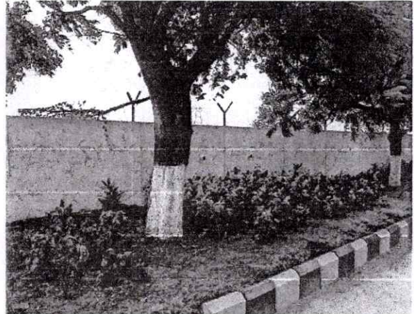
Compound Wall Snap-2
