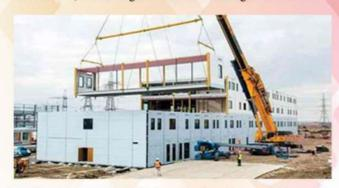
It also offers strong sustainability benefits, from fewer vehicle movements to less waste. By using this method with up to 70 percent of a building produced as components, it allows a move towards "just in time" manufacturing and delivery.
