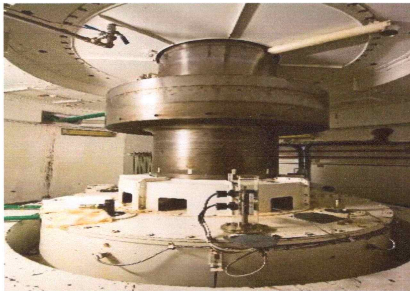
Fig. (a) Srisailem Francis turbine
