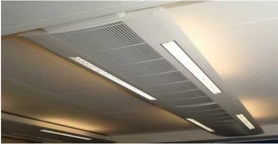
3.3: Radiant cooling panel attached to ceiling
