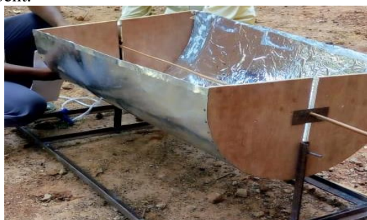
Fig-2. Fabrication of solar parabolic trough collector
