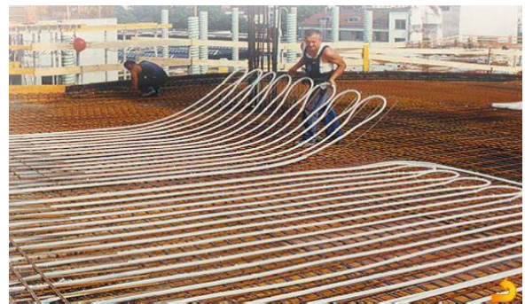
Figure 3.2: Laying of PEX pipes in Slab
